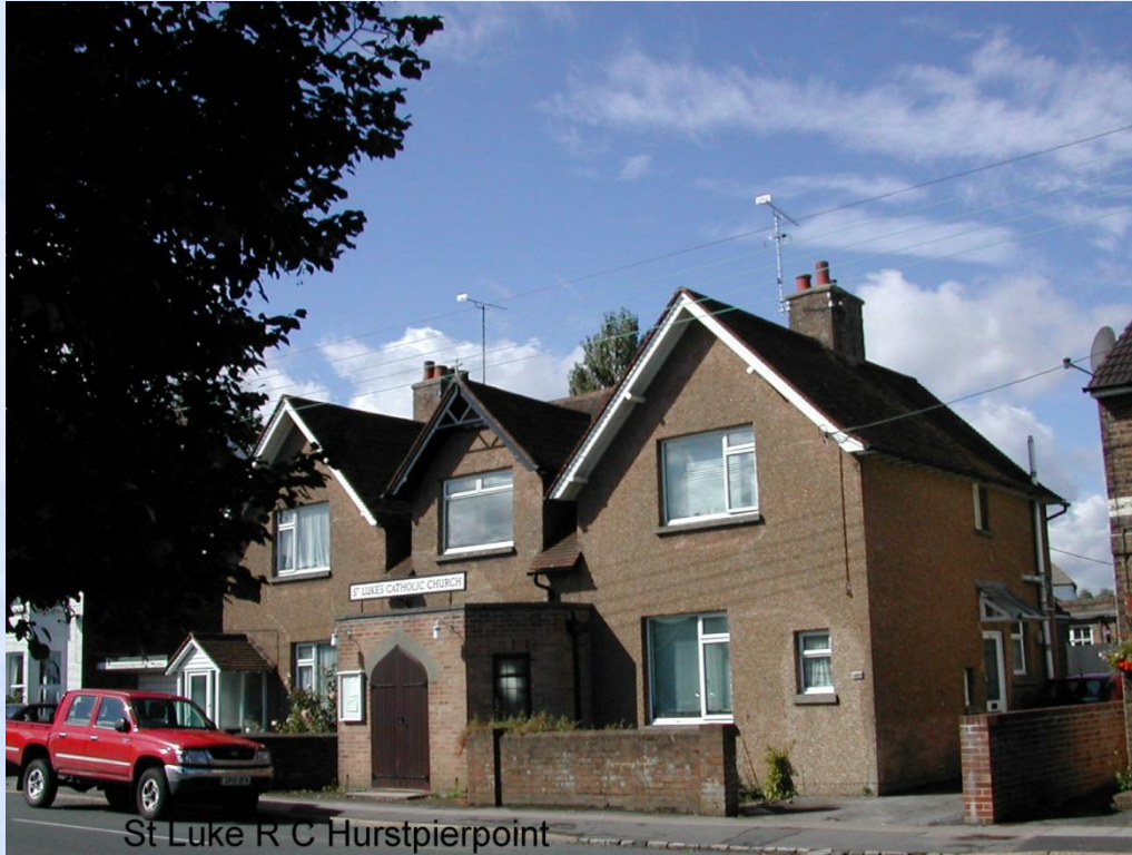
Roman Catholic St. Luke's, Cuckfield Road
