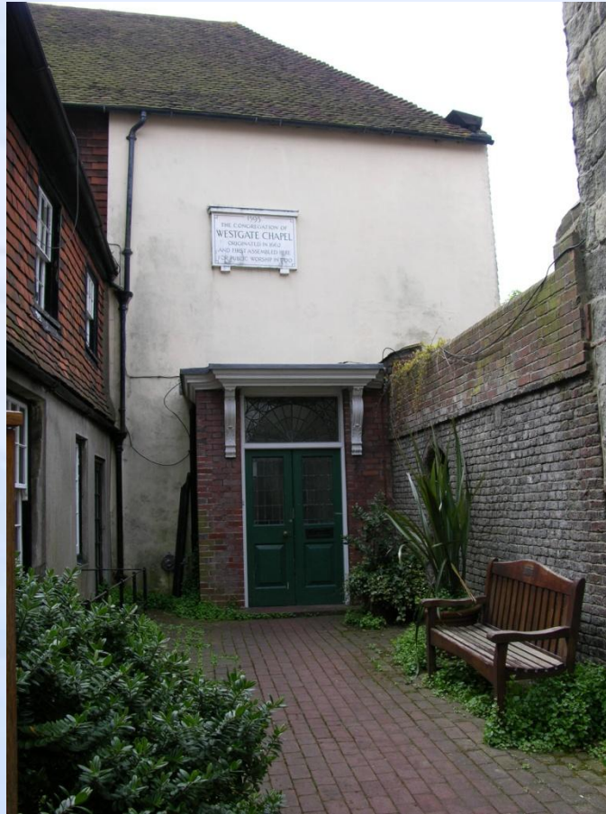
Westgate chapel Dissenters, a Building, High Street (registered for worship 1824)
